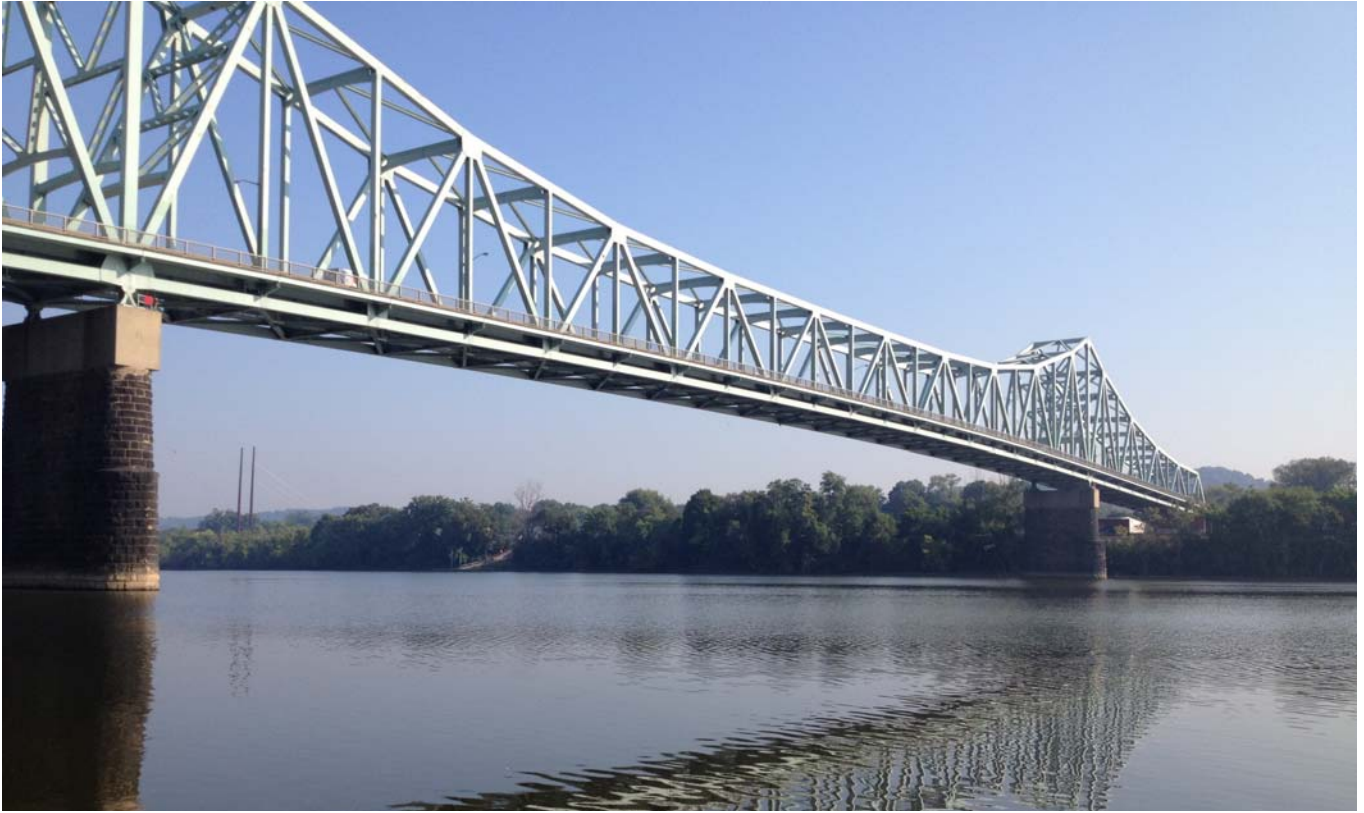
Sewickley Bridge from Riverfront Park
